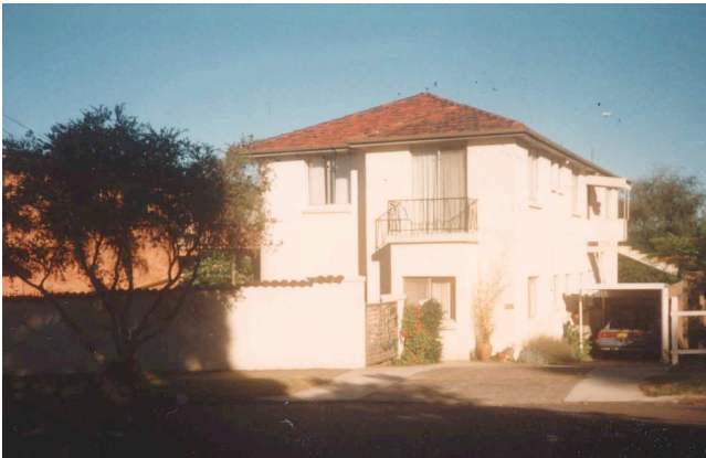
137 Greenwich Road, Greenwich, NSW.
