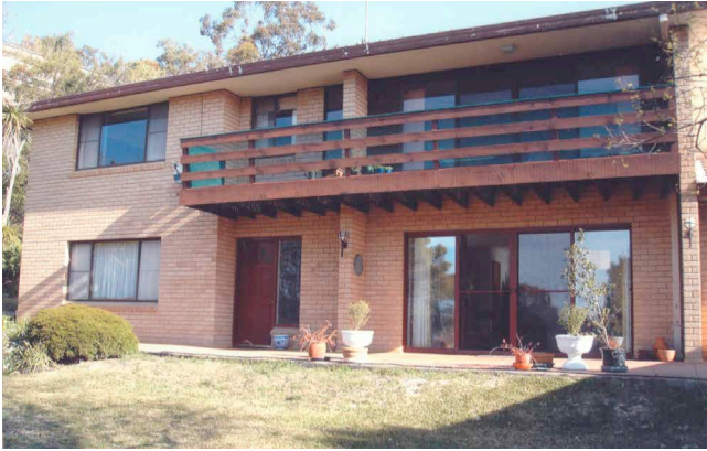
78 Lonsdale Avenue, Berowra Heights, NSW.
