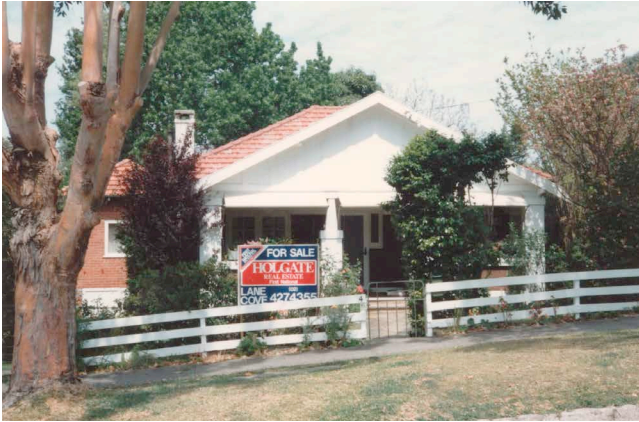
4 Kingslangley Road, Greenwich, NSW.
