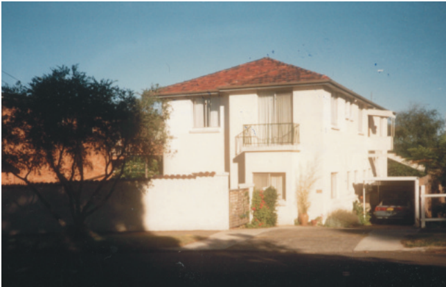
139 Greenwich Road, Greenwich, NSW.
