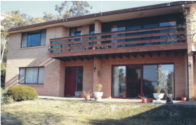
78 Lonsdale Avenue, Berowra Heights, NSW.
