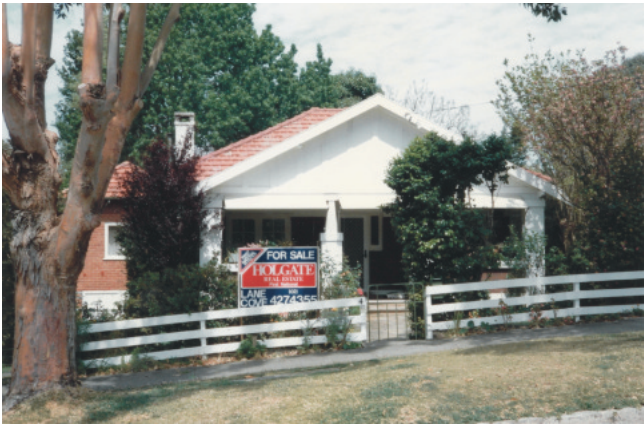
4 Kingslangley Road, Greenwich, NSW.
