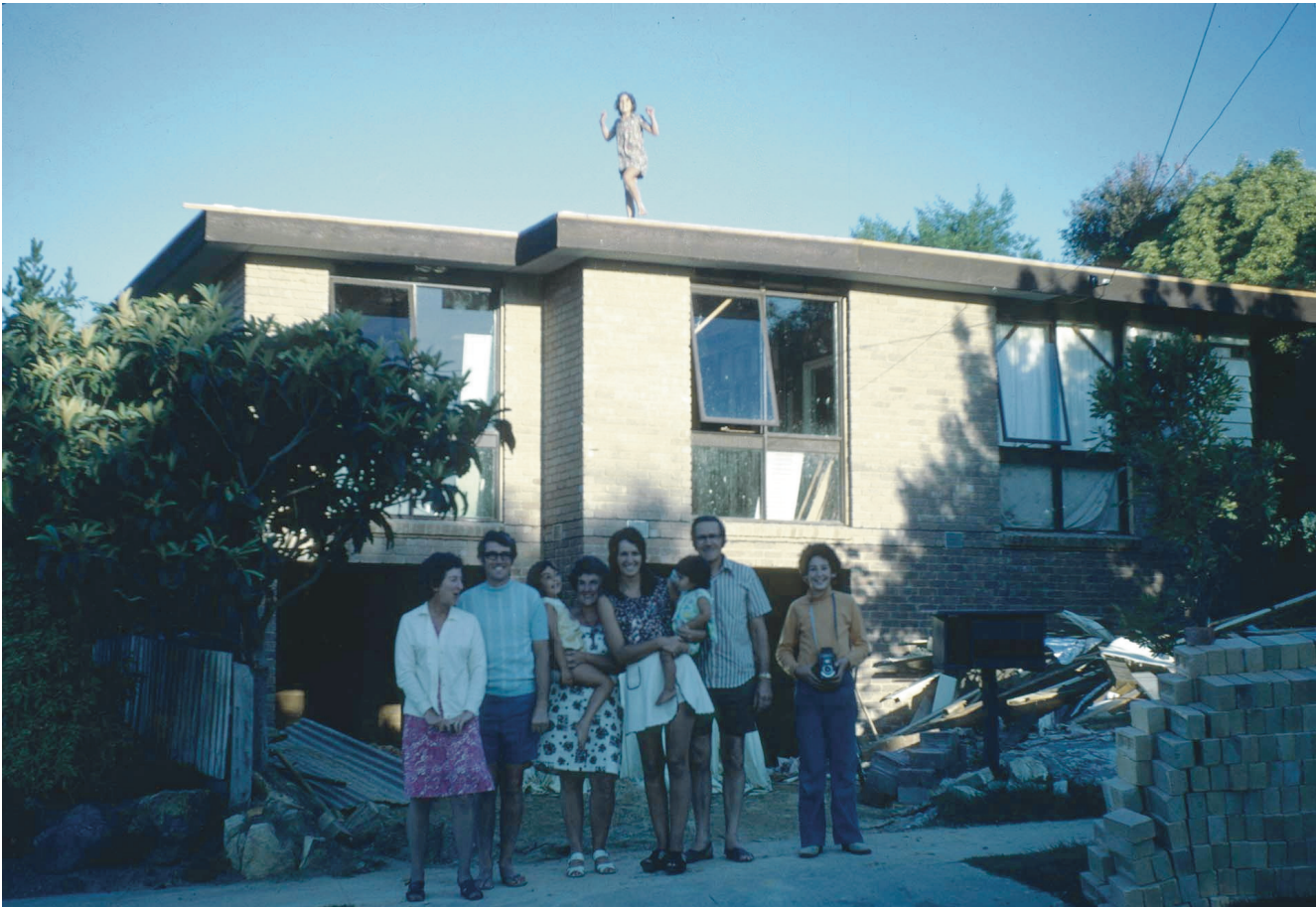
16 Glendowan Road, Mount Waverley, Vlctoria, 1973. Far left: Shirley; far right: Matthew; on roof: Jenny.
