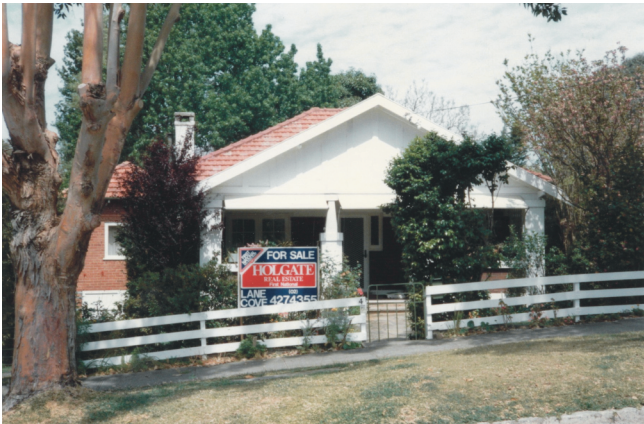
4 Kingslangley Road, Greenwich, NSW.
