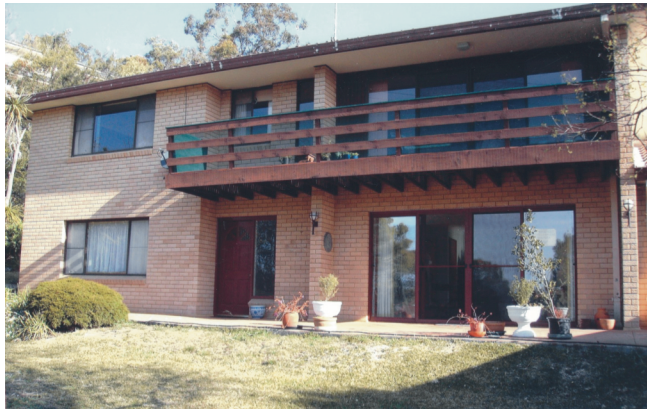
78 Lonsdale Avenue, Berowra Heights, NSW.
